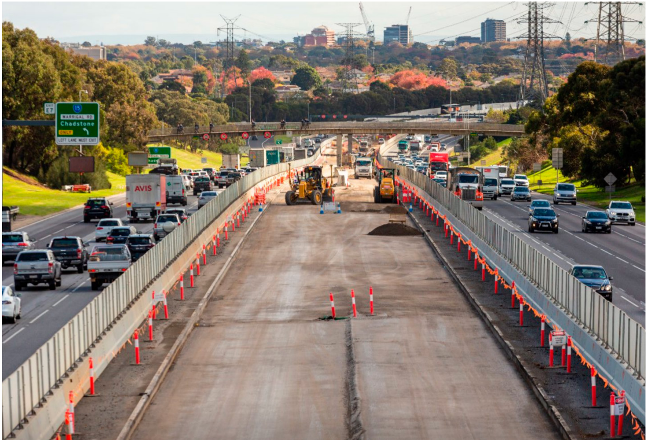
Figure 2: New lanes of the Monash Freeway between Huntingdale and Warrigal Road
