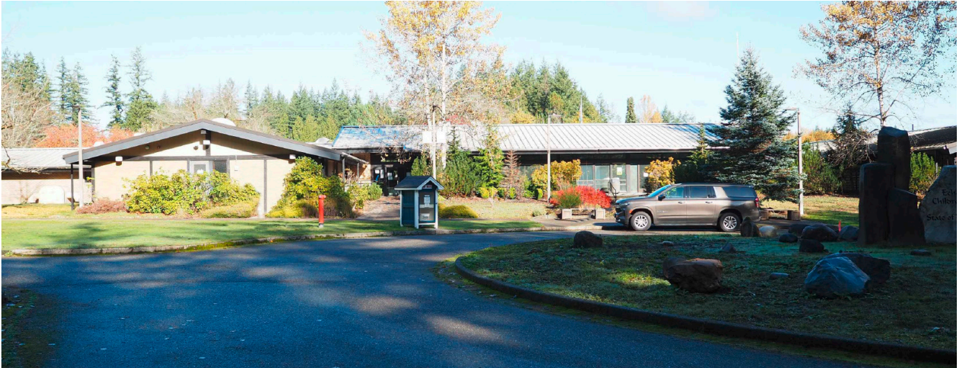
Echo Glenn facility
